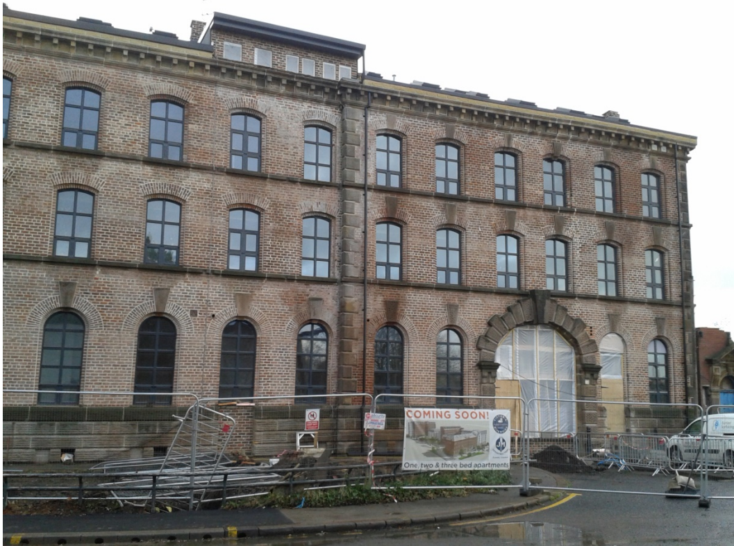
Photo 1: Victoria Mill, Holbeck, has been largely converted to residential use.
