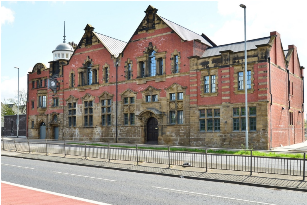
Photo 2: York Road Library, Burmatofts, has been converted to a gym.
